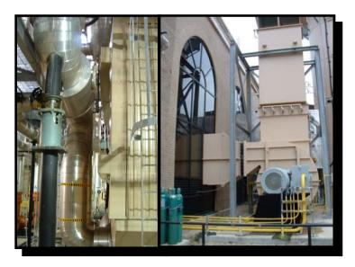
heat economizer, VFD driven force draft fan, etc.). A new continuous emissions monitoring system (CEMS) and a new 8" gas supply line were provided. The existing 200 feet tall concrete, historical stack was refurbished.
